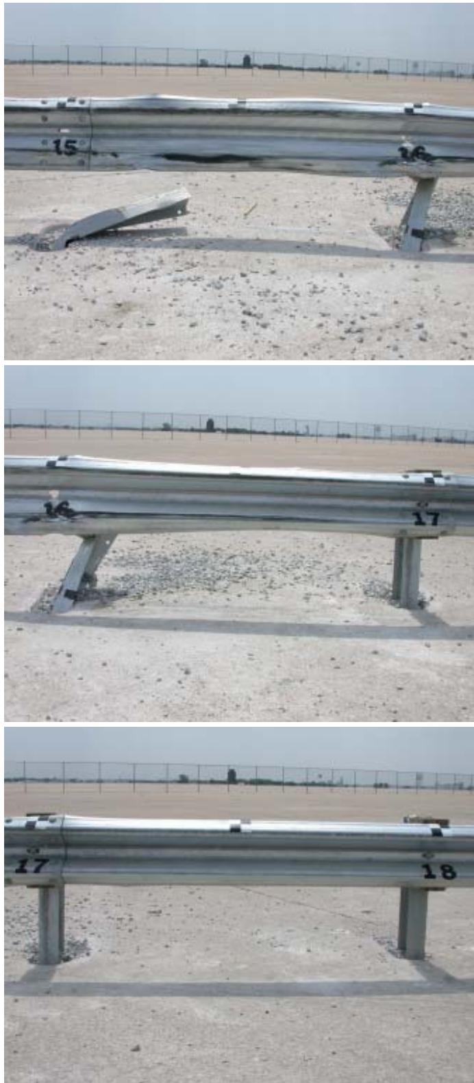
Figure 47. W-beam Guardrail System Damage, Test PR-1
