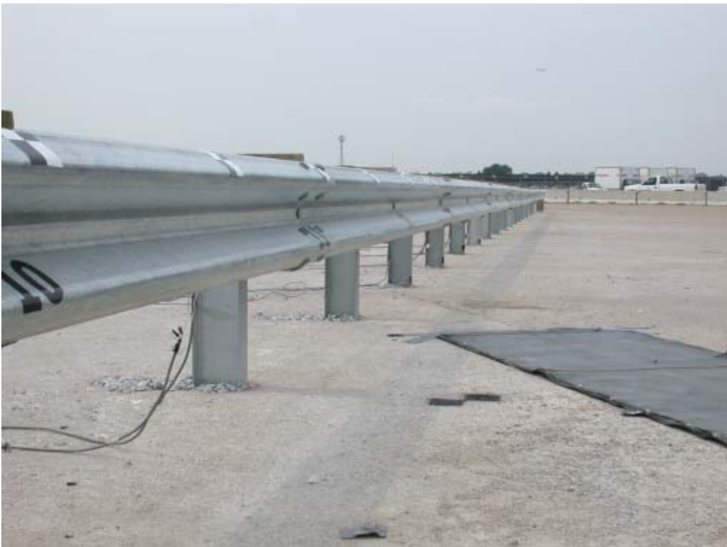
Figure 33. W-beam Guardrail Attached to Posts in Rock
