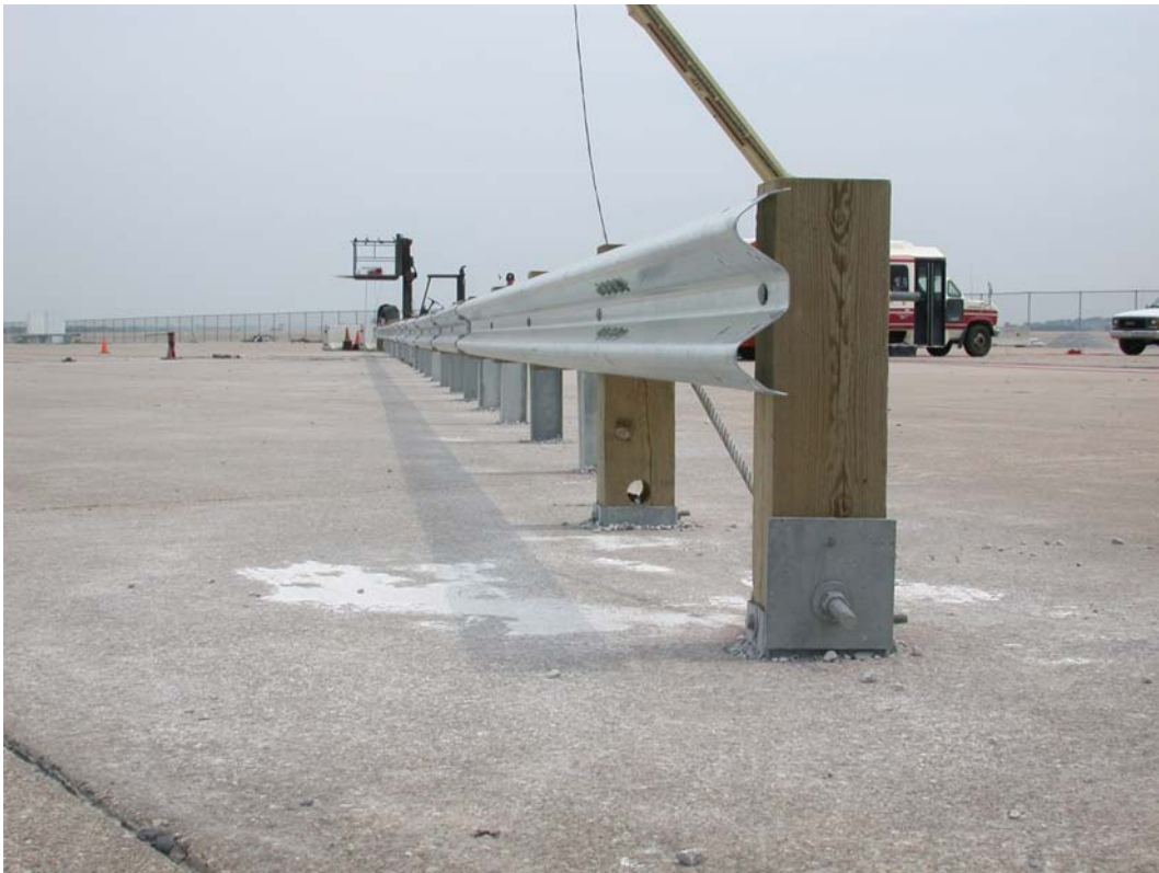
Figure 32. W-beam Guardrail Attached to Posts in Rock
