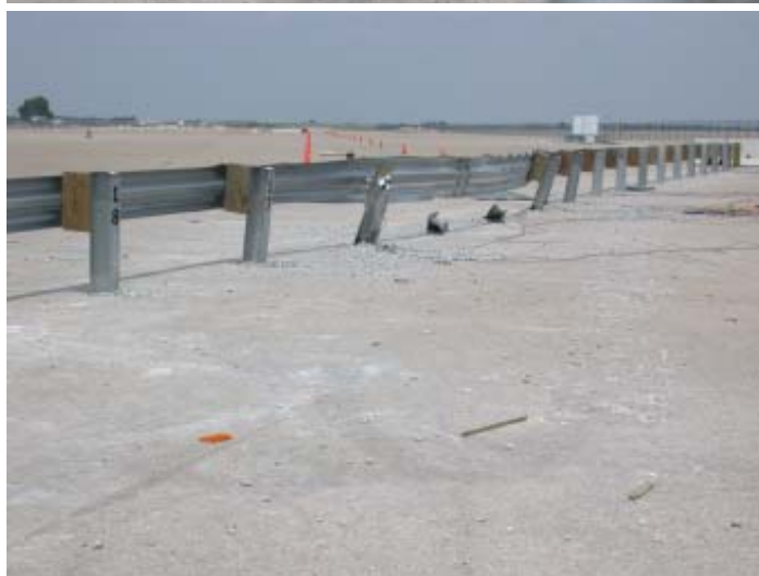
Figure 44. W-beam Guardrail System Damage, Test PR-1
