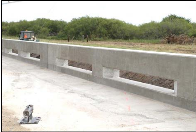
Figure 3.37 TxDOT T224 MASH TL-5 Bridge Rail System (10) .
