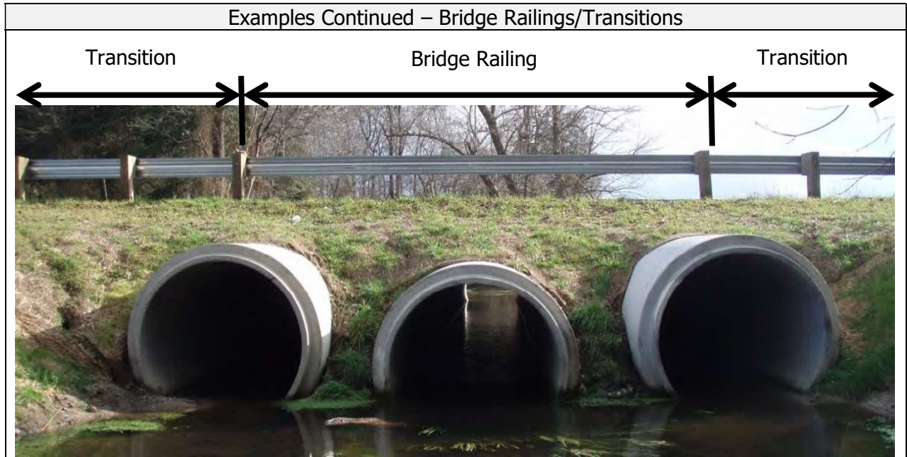
Figure 12. Metal bridge railing and transition for long-span application. (Source: Delaware DOT)
