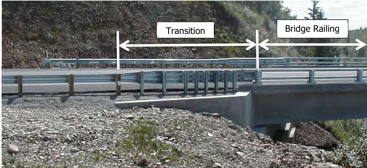
Figure 11. Metal bridge railing and transition. (Source: Alaska DOT)
