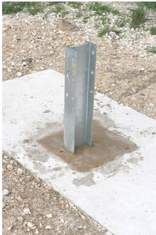
Figure 18: Leaveout with two-sack grout prior to test B1.
