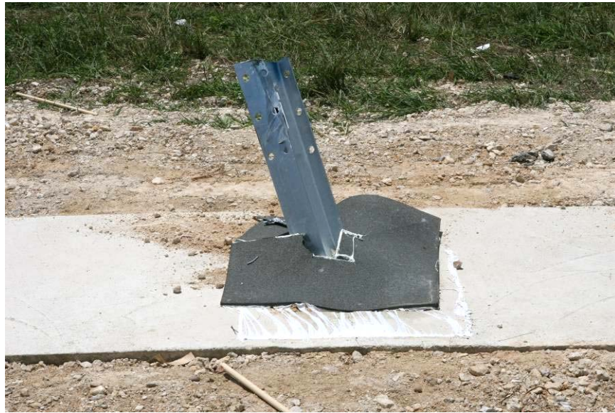
Figure 12: Post with flat mat after test B5.
