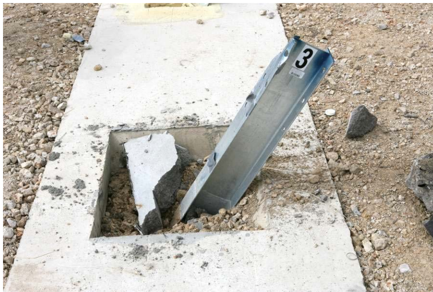
Figure 23: Post in full-strength unreinforced concrete wedge after test B3.
