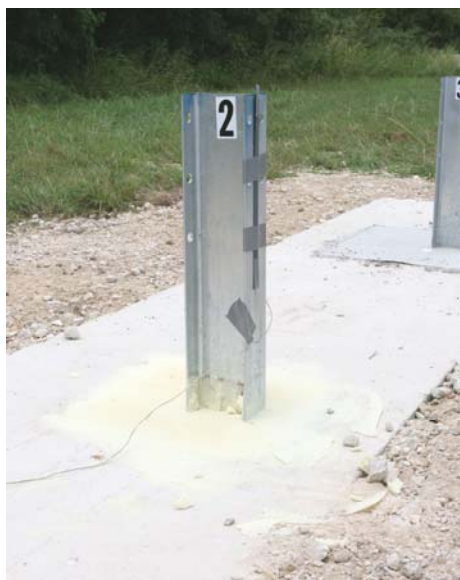
Figure 20: Post in two part urethane foam prior to test B2.
